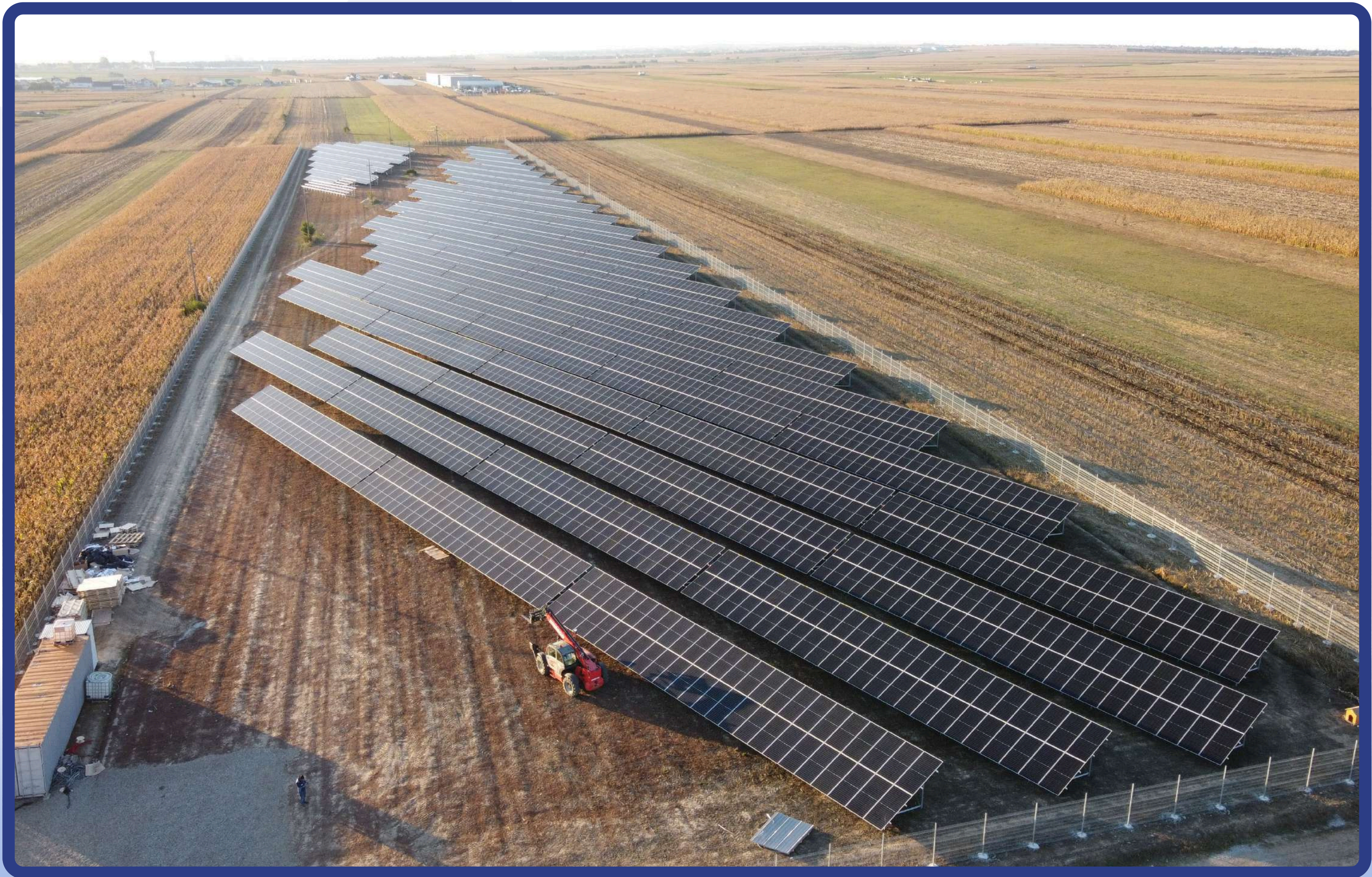
COLINA SOLAR - Veresti 2 MWp Structura fixa ALUMIL- Sep 2023 - Nov 2023
