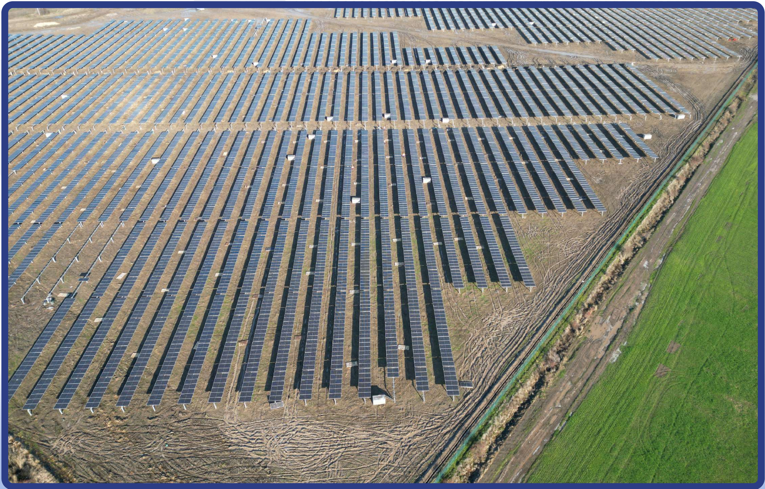
Alerion Italia- Alexandria 13 MWp Valmont 1P tracker structure - Oct 2022 - Mar 2023
