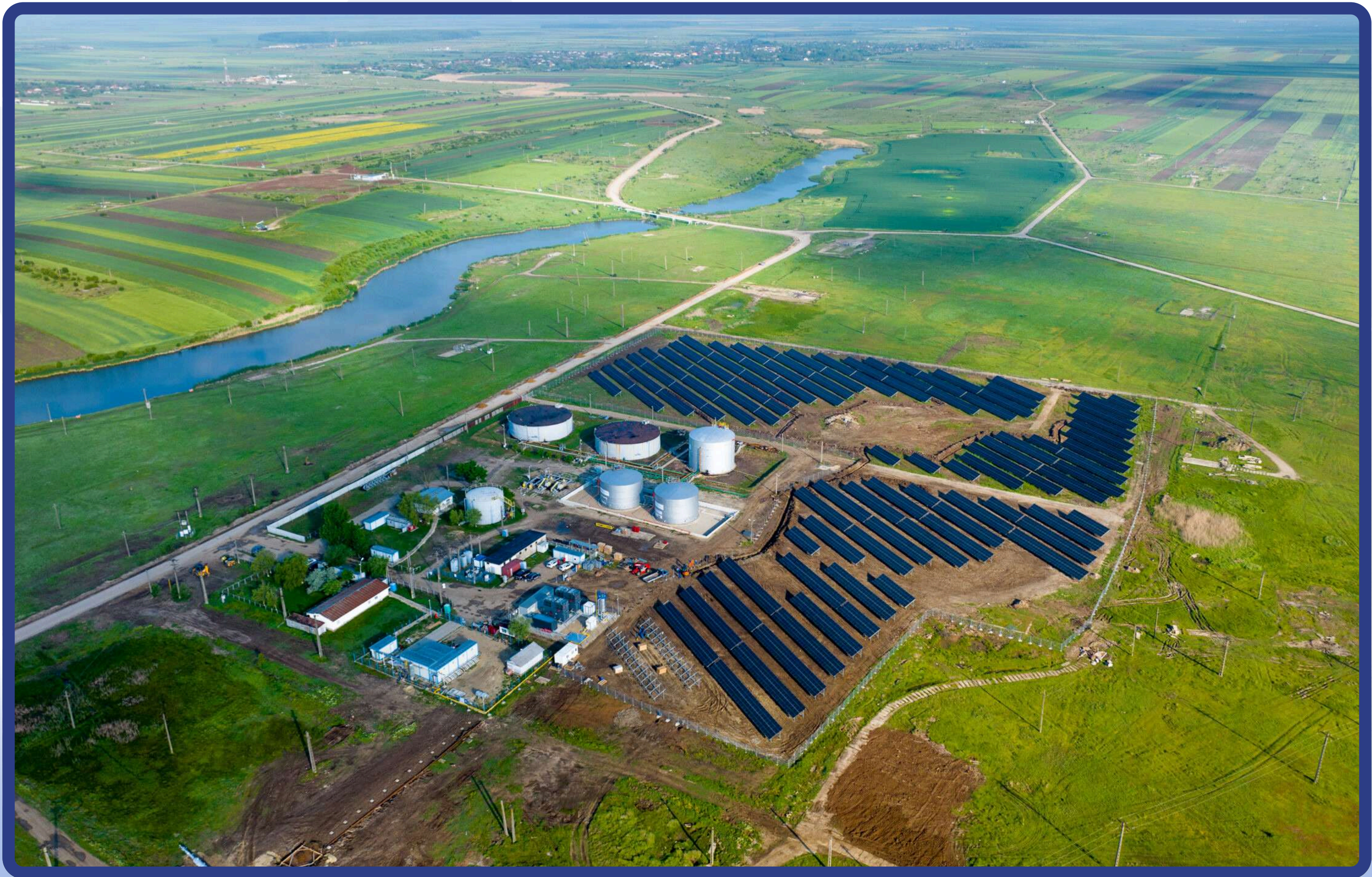
Petrom - Cosmesti 2 MWp Structura fixa 2P- Oct 2022 - May 2023
